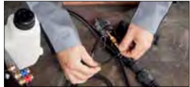
4. Mount the shrink hose for insulation.
