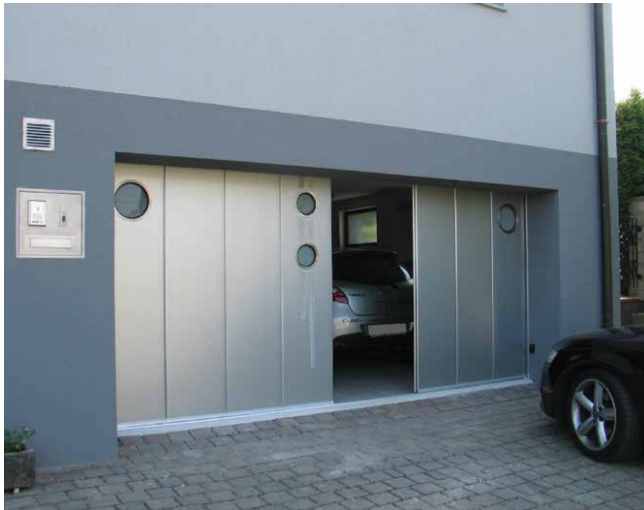
The Side Sliding Sectional Door
