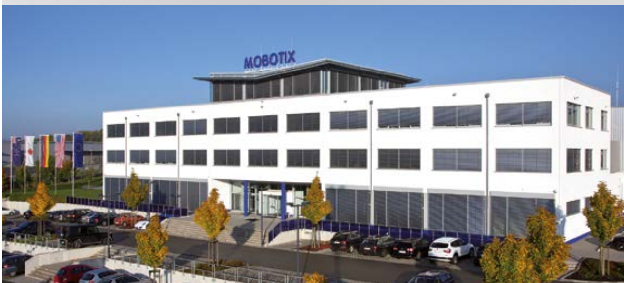
MOBOTIX Headquarters Langmeil, Germany
