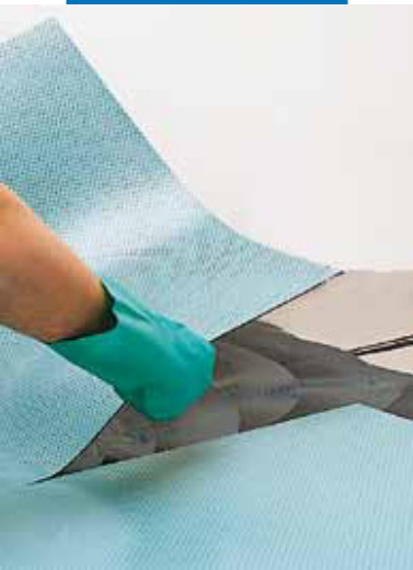
Laying conductive PVC tiles
