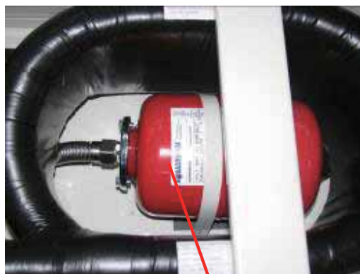
Expansion gas tank Fig. 7
