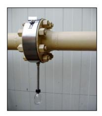
Leak detection and fire protection nipples for fixing stainless steel drainage pipes are optional.
