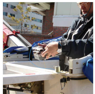
On a Bucket Truck
