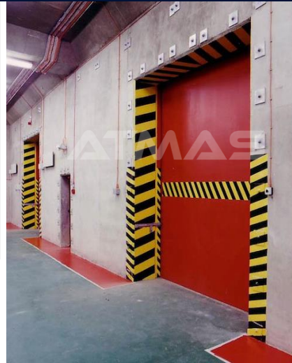
Blast doors with concrete insert
