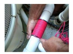
5.) Route the loose end of the signal cable back to the power unit. Trim the cable to length. There may be several feet of unused wire. This extra wire was included in case the control box was mounted several feet away from the return line.
