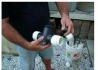
2.) If the pipe size where the flow-cell chambe is being installed is 1 ½", glue the two reducer bushings (2" x 1 ½") into the male adapters. This step is not necessary if installing on two-inch pipe.
