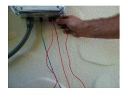
6.) Carefully strip the outer plastic shield from the end of the signal cable, leaving about 1/4" to 3/8" of bare cable. Twist the bare cable and insert the end into the unused receptacle post on the power unit. Tighten the receptacle post. Make sure all the threads of the signal cable go though the terminal hole.
