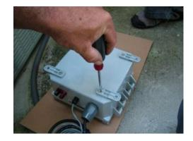
2.) Mount the microprocessor control box to the wall allowing for the power cable wire to reach the source of power; the electrode wire to reach the electrodes; and the **ScaleBlaster** signal cable to wrap around the pipe - also on the return line. Use proper anchors and screws to mount on the surface (wood, stucco etc.).
