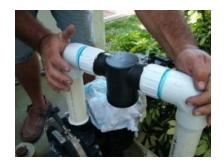
6.) Seat the "O" ring in the electrode jar and screw into the black flow-cell chamber by using your hands. No Teflon tape or wrench required!
