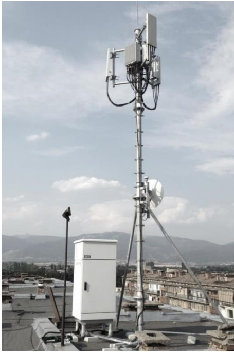
Air conditioning Double walls
