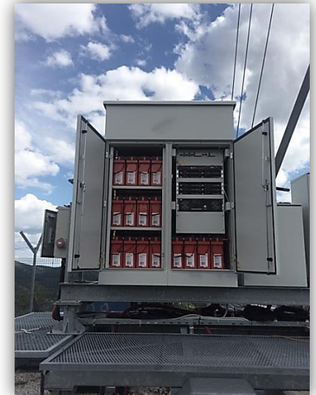
Outdoor cabinet COOLRACK, double walls, A/C, 19" free space for clients equipment
